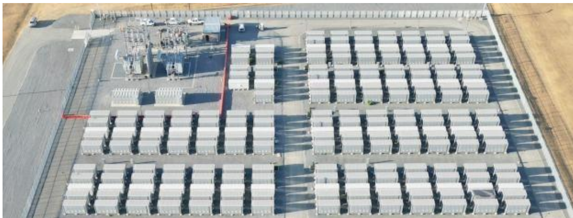
2.3.4 Fig. Example of site development within the BESS area (photo source: BEIConstruction.com).
